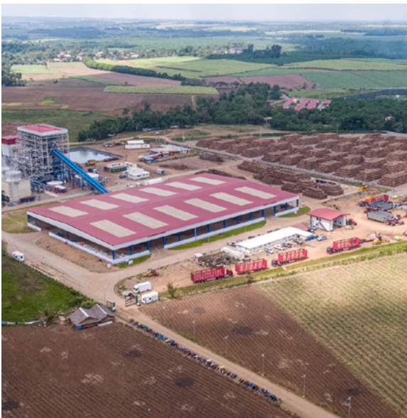
Biomasse-Kraftwerk North Negros Biopower, Philippinen
